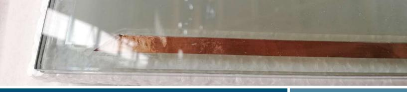
Switchable laminated glass that changes light transmittance instantly from a white translucent opacity to visible transparency. This transformation is possible with the combination of a unique liquid crystal interlayer lamination and electricity.
